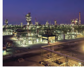
GASCO HABSHAN PROJECT (United Arab Emirates)
