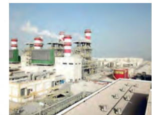
UMM AL HOUL POWER PLANT (Qatar)
