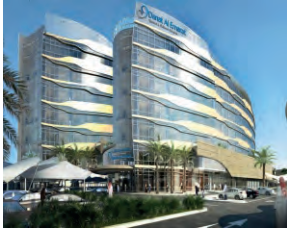
DANAT AL EMARAT HOSPITAL (United Arab Emirates)
